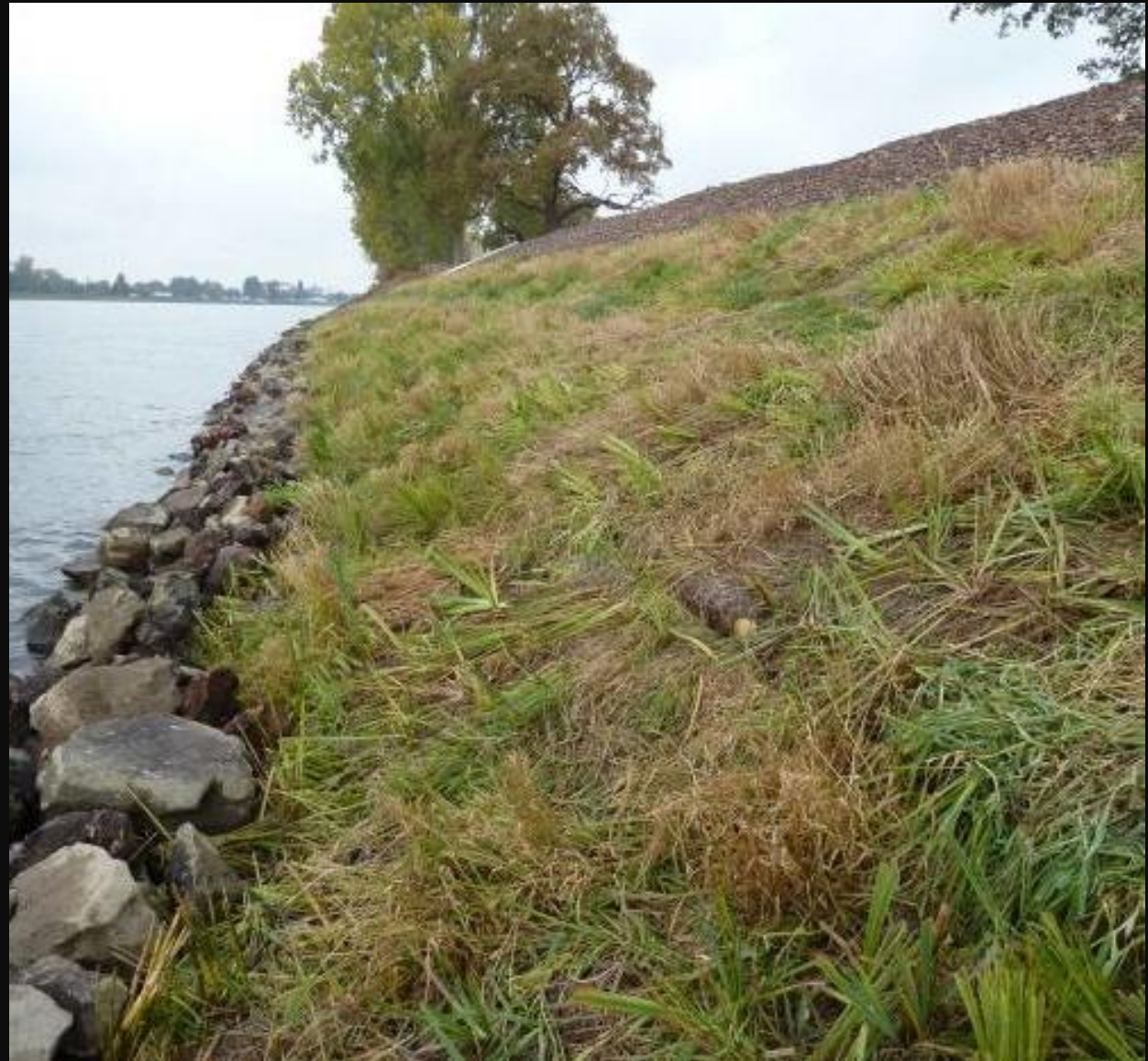
Figure: Reed gabions on the Rhine River (PIANC WG 128)
