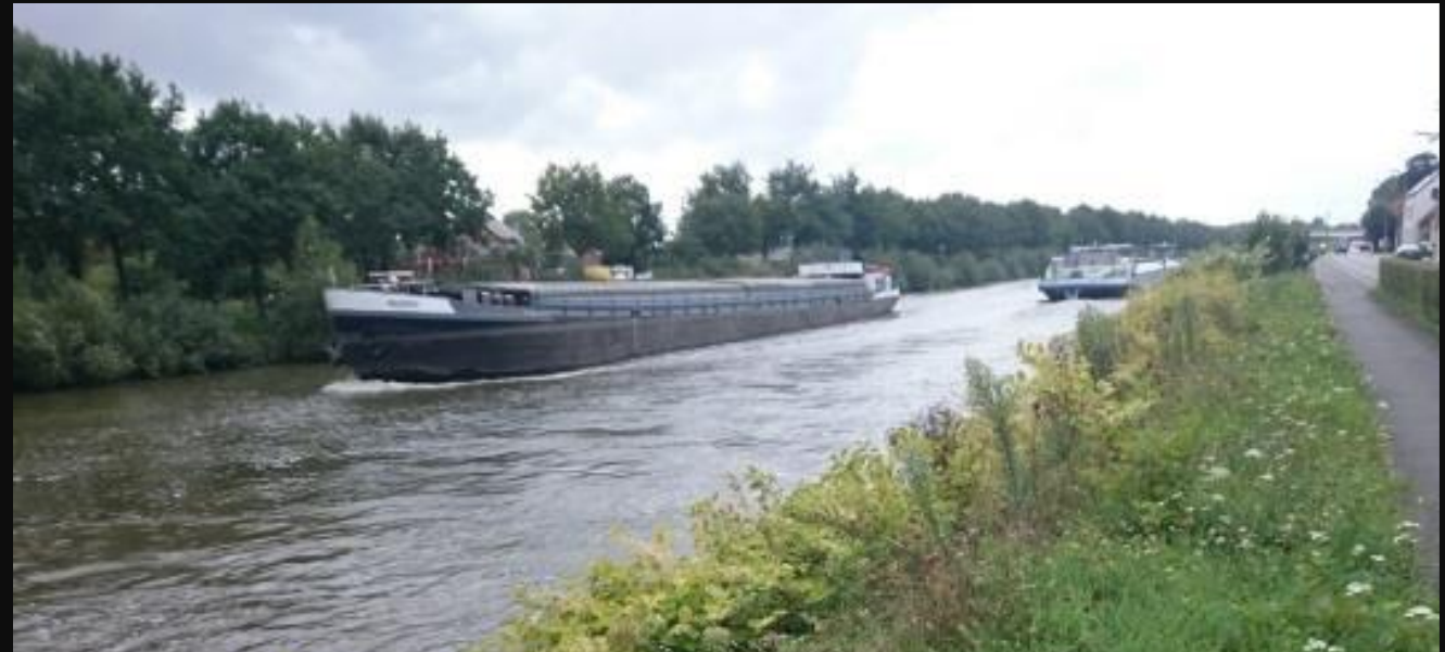
Figures: Permeable palisades with reed planting close to Essel Town, Germany (Berhard Söhngen), Shallow-water zone protected by parallel dam for the Canal Ghent–Bruges, Belgium (Jeroen Verbelen)
