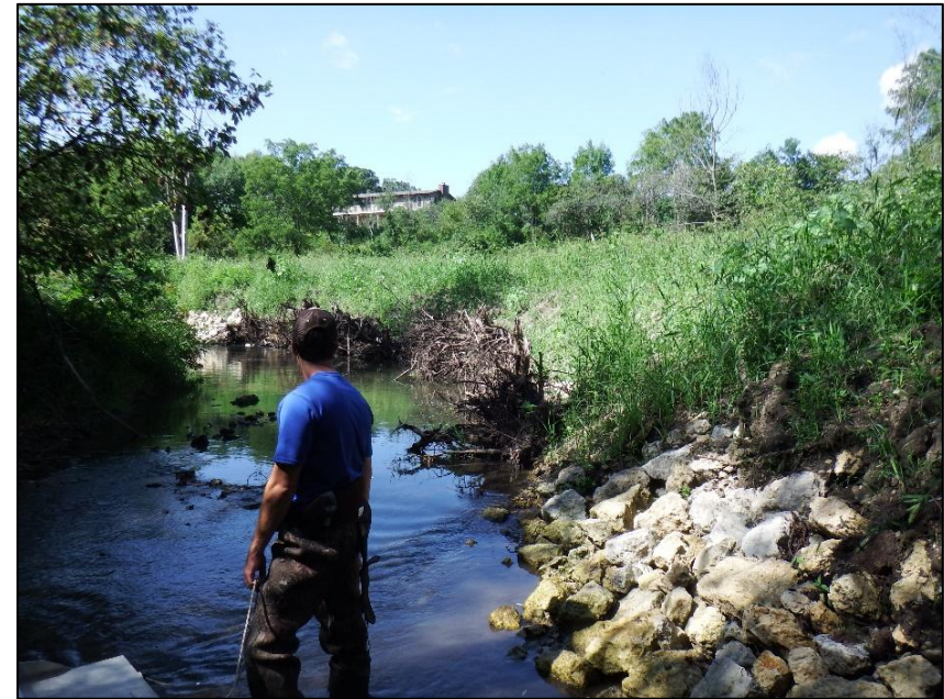
Figures: Wattle Fence at Gernsheim, Rhine (WG128) and root wads with longitudinal peak stone toe protection (Chris Haring)
