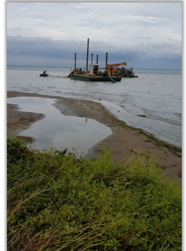
Placing dredged material from the navigation channel in the wetland. (Photo USACE Detroit District)
