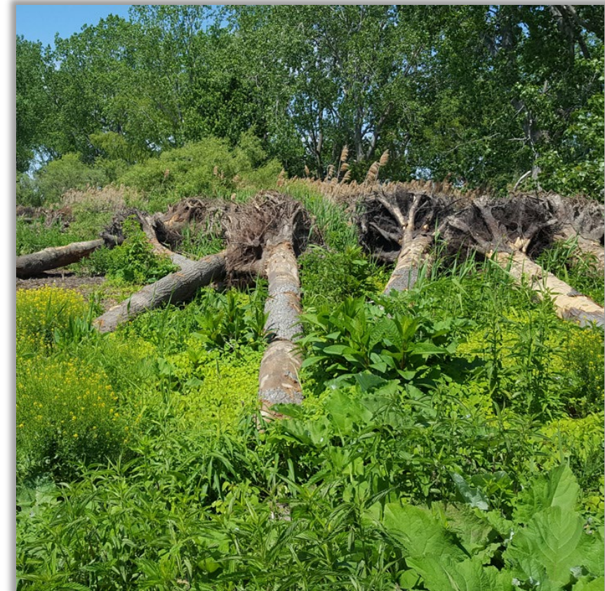
Root wads for anchoring to the lake bottom as a wave break. (Photo by Keith Kropfreiter, USACE Detroit District)
