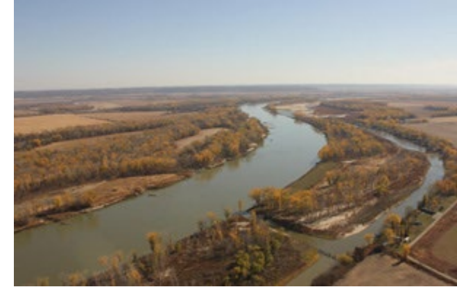
Preconstruction view of Deer Island in 2012. (Photo by Dave Crane, USACE Omaha District)
