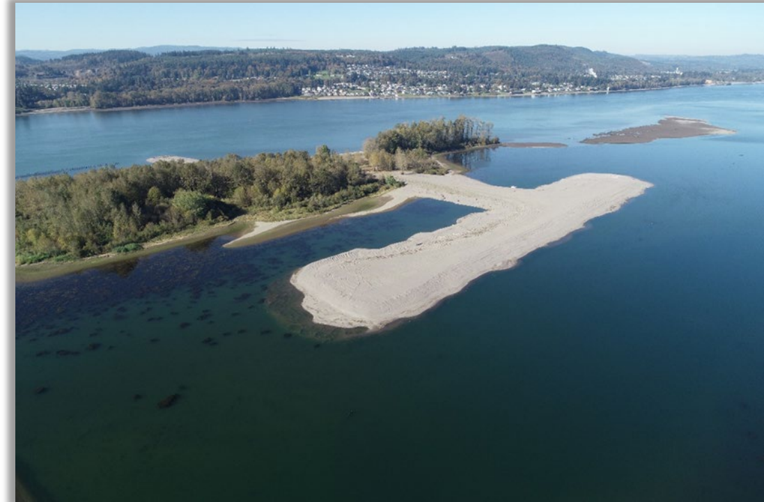
Woodland Island downstream feature constructed in fall 2020 from 200,000 cy dredged sediment and subsequent grading for restoring riverine habitats (Columbia River Estuary Study Taskforce).
