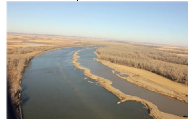
Center of the project site during construction. (Photo by Dave Crane, USACE Omaha District)
